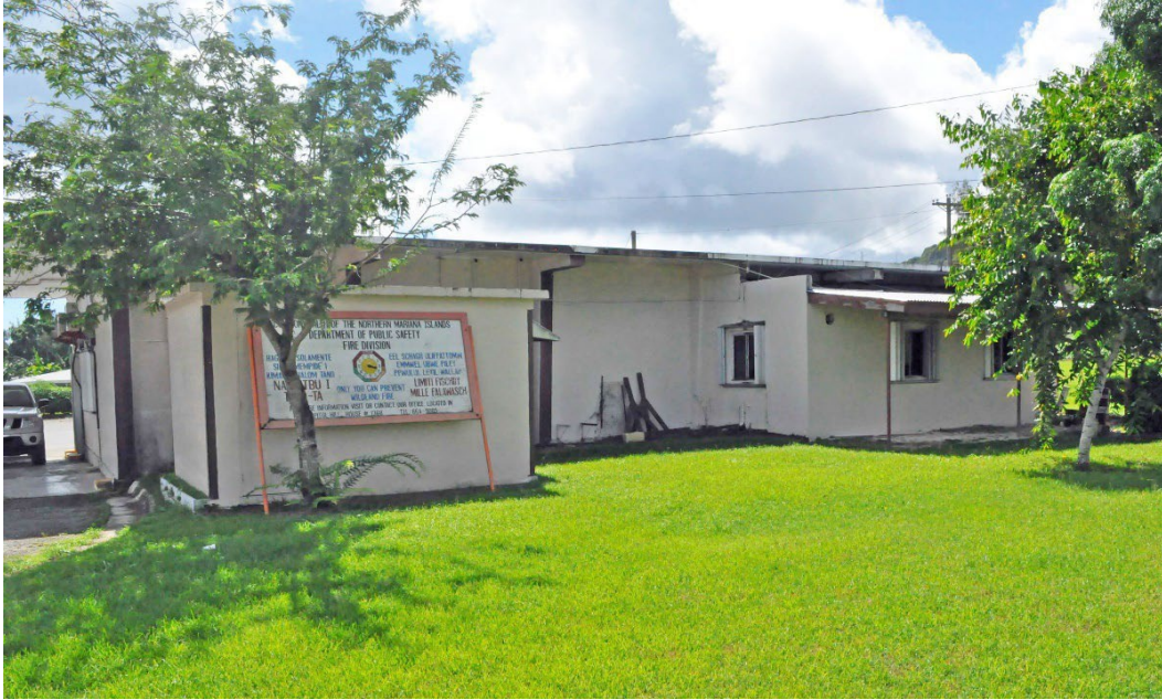
Figure 123. West elevation of Feature 6. Note concrete block extensions to the original building.
