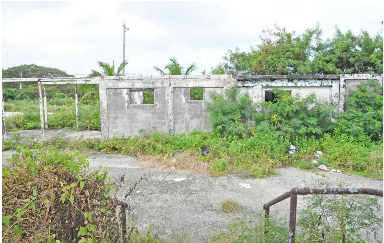
Figure 199. Feature 125, a generator building for the original NTTU mess/club. It was expanded by the TTPI.
