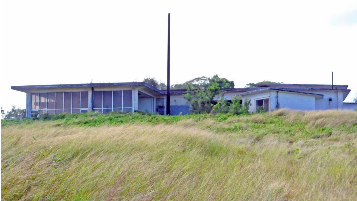
Figure 192. Feature 124 north elevation view showing CNMI-era expansion.
