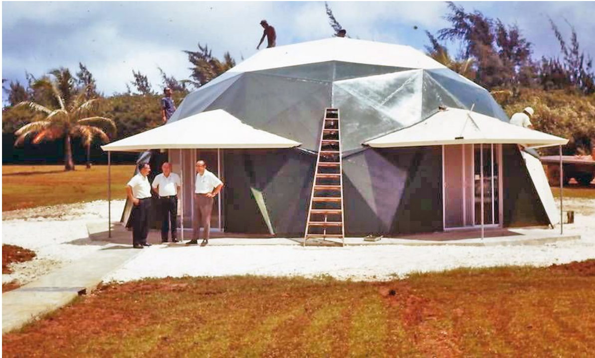
Figure 143. Feature 18, a TTPI-era geodesic dome while under construction circa 1967.
