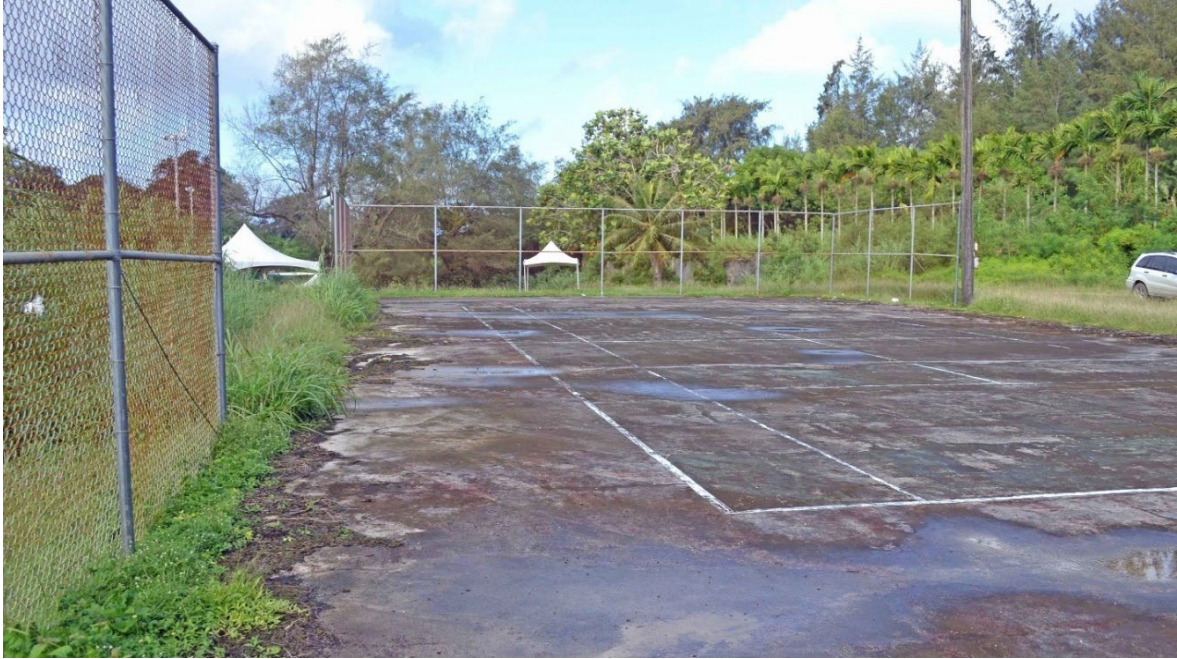
Figure 145. Feature 21, a NTTU-period tennis court with chain link ball stops at both ends.
