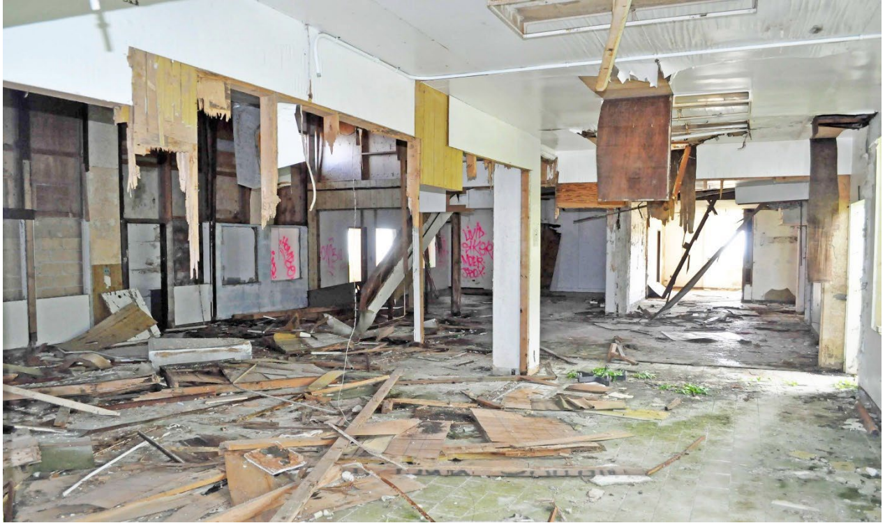
Figure 196. Original bar and dance area of Feature 124. Plywood represents post-NTTU ceiling and partitioning.
