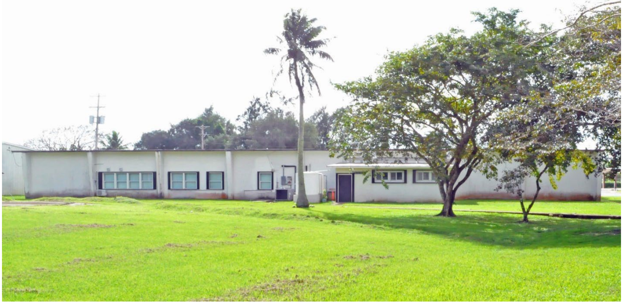
Figure 135. West elevation of Feature 11a. Windows and concrete block extension are not original.
