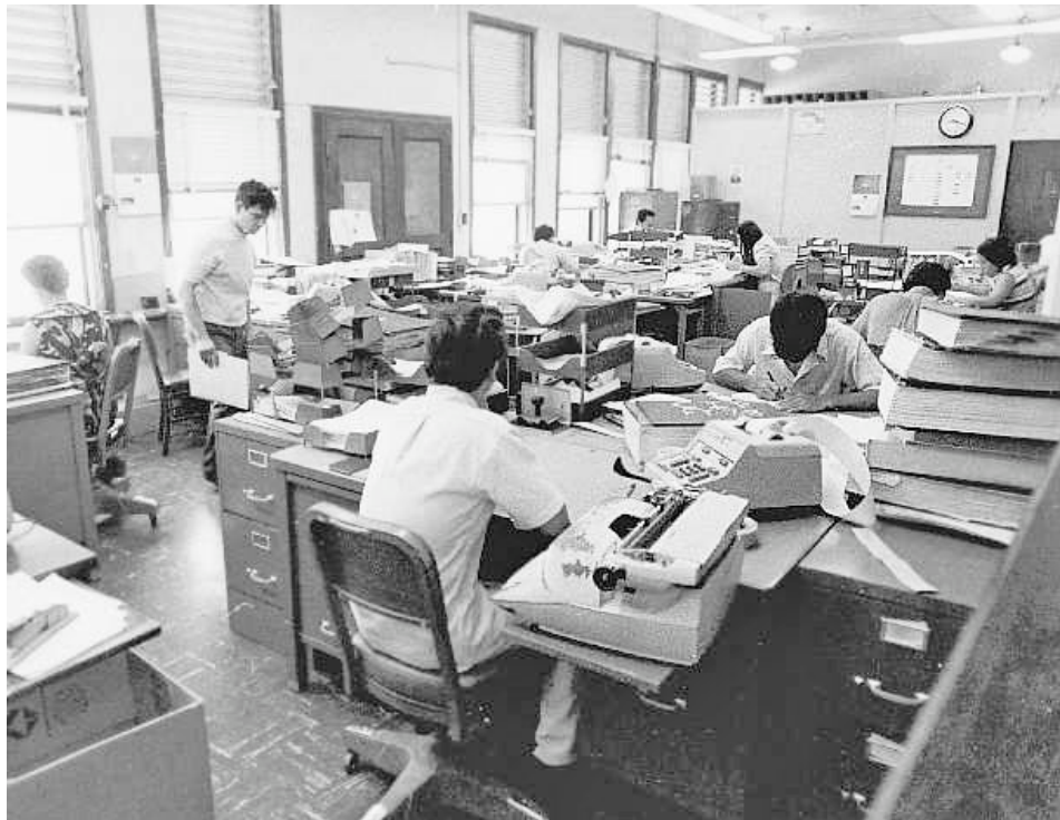
Figure 85. TPI finance office on the first floor of the headquarters building, circa the early 1970s. Note original windows and floor tiles.
