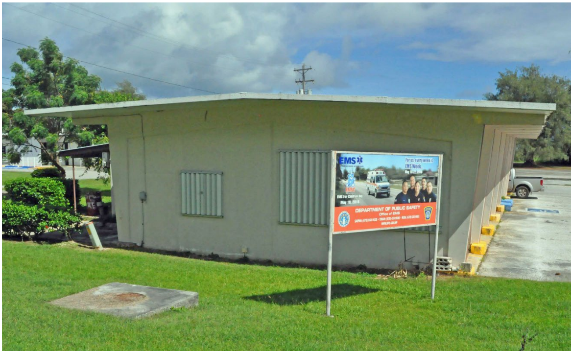
Figure 124. South elevation of Feature 6. Windows, which are not original, have been equipped with metal storm shutters.
