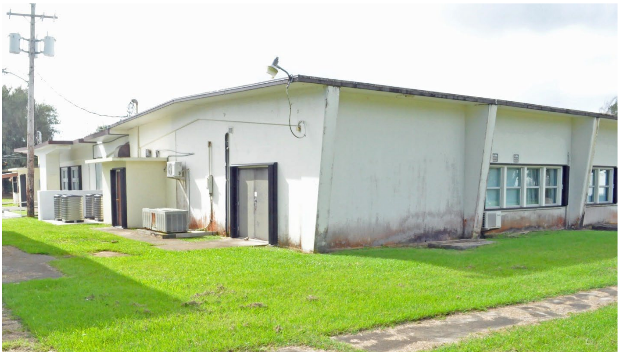
Figure 136. Northwest corner of Feature 11a showing original tapered columns and gently sloping gabled roof. Also visible is a small cinder block extension. Windows at right are not original NTTU period construction.
