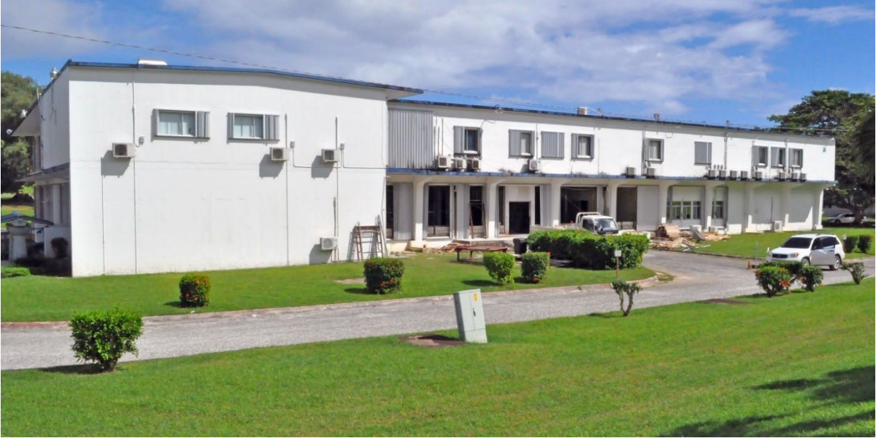
Figure 107. Southwest elevation view of Feature 1. This photograph was taken during renovation work to install an elevator to the second floor. Note exposed columns and beams that were added to support the new office space on the second floor in the late 1980. Original pane and louver windows have been replaced on this wing.
