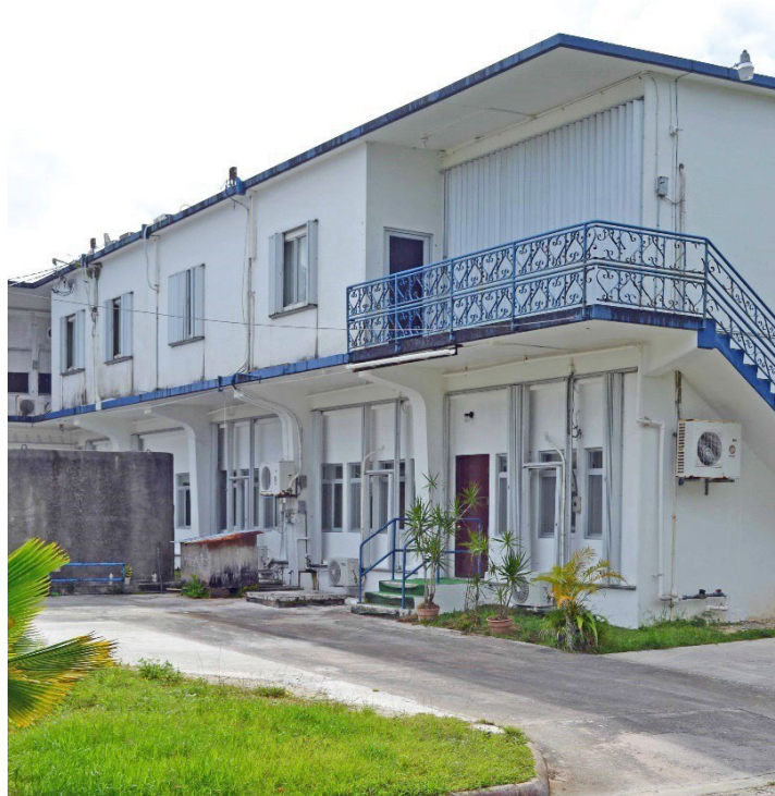
Figure 110. Feature 1, second floor office extension and stairway built in the 1980s.
