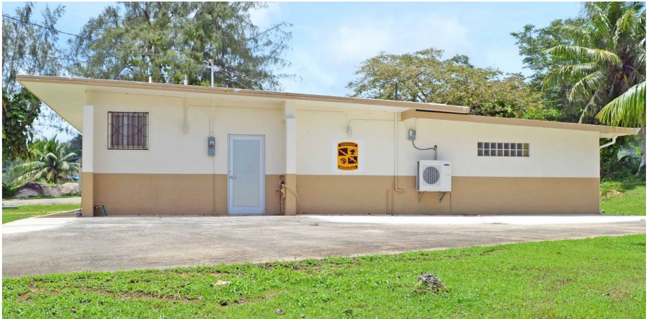
Figure 169. Feature 119 showing sizable concrete block extension (at right) and window alterations.
