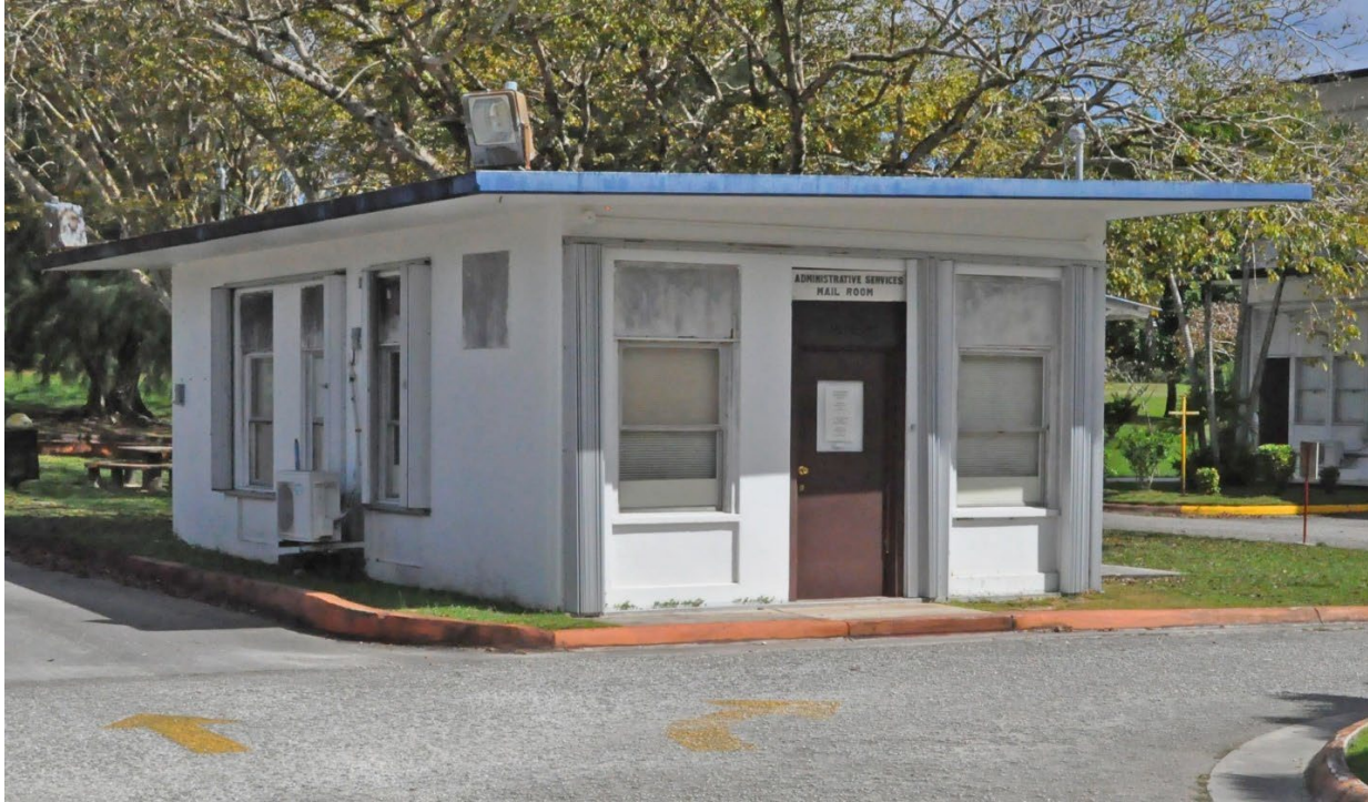
Figure 115. Feature 2 exhibiting original pane windows (with louvers covered). Note metal storm shutters.
