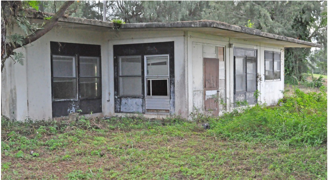
Figure 153. Feature 50 showing dining room/porch details. Note original aluminum louvers on bottom of the two-window set. Others are also present but covered with painted plywood. Original outdoor light fixture is also present.
