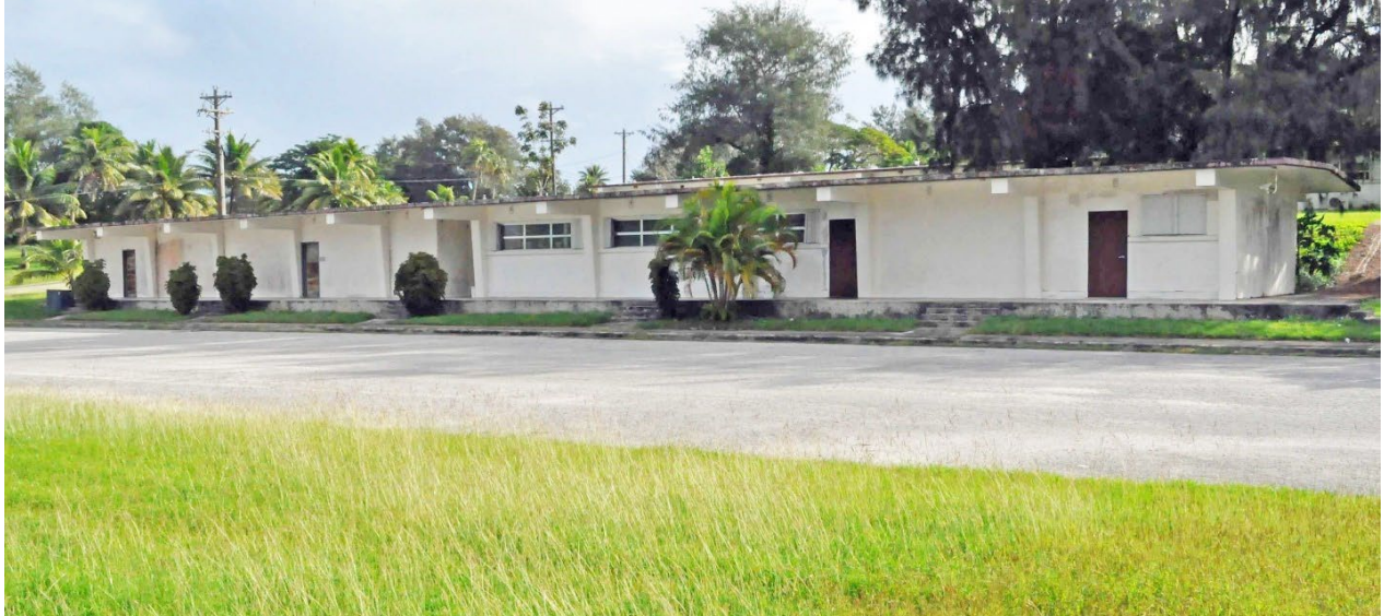
Figure 178. West elevation of Feature 74, Recreation Building B. Its original windows are no longer extant. Note tapered beams and columns and the covered walkway through the mid-point of the building. Feature 72 is in foreground.
