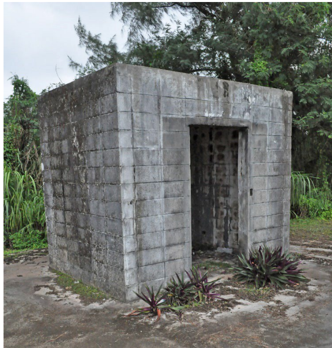
Figure 128. Concrete block room located at the east end of Feature 9. It originally functioned as a vault.
