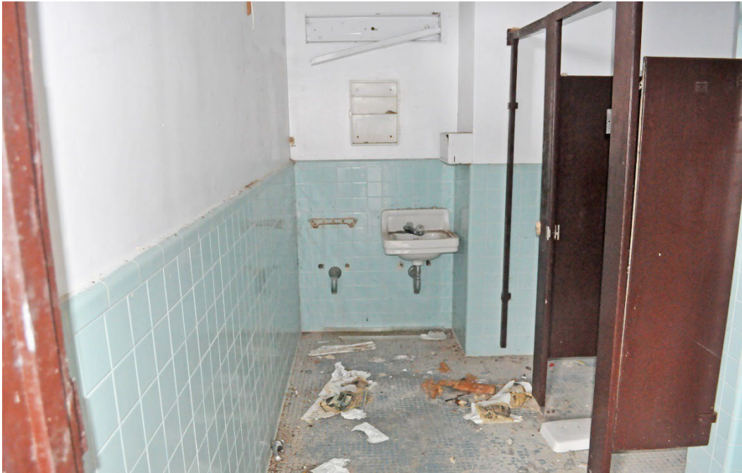
Figure 197. Bathroom in Feature 124 showing original tiling, lavatory sink and stall partitions.
