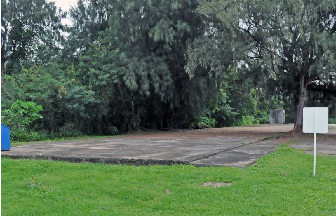
Figure 127. Concrete slab of Feature 9, a TTPI-era government office building. Looking northeast.
