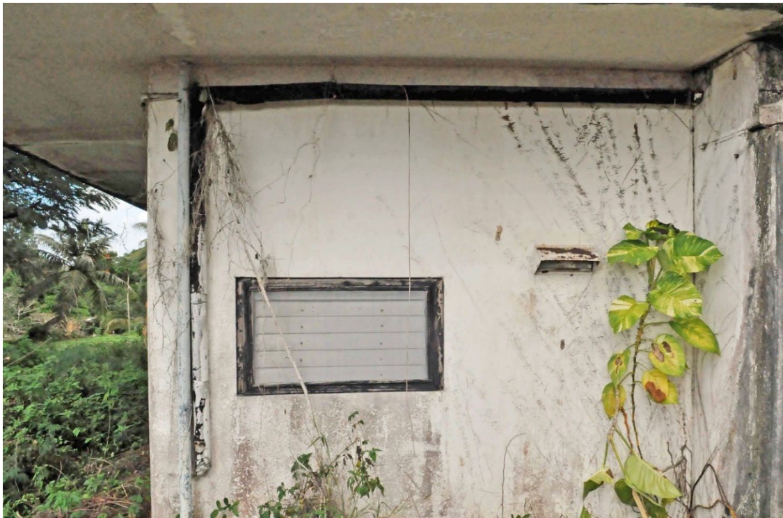
Figure 156. Feature 50 with original louvered kitchen window. Also note stove vent and insulated water piping that runs on outside of wall.
