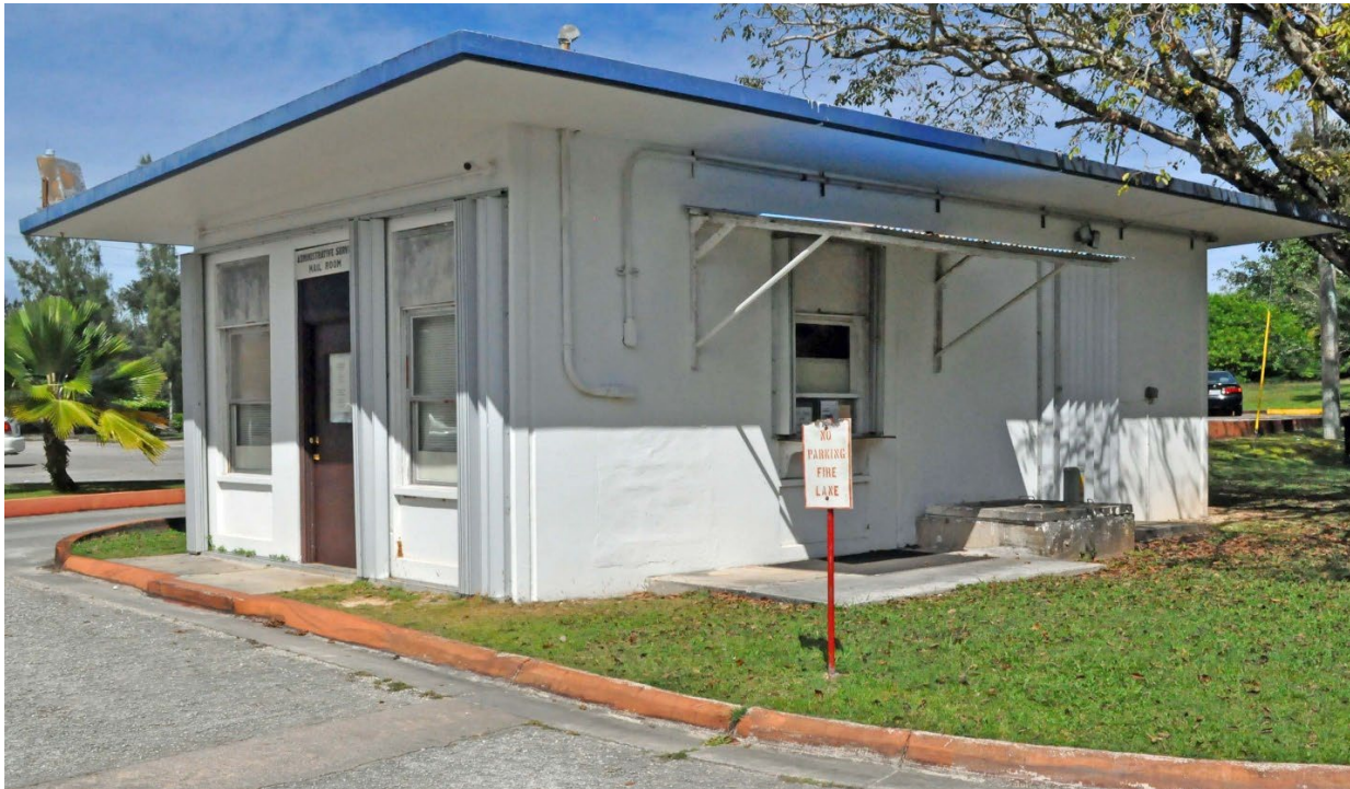
Figure 116. Feature 2, north elevation. This elevation has had most of the original windows blocked in.
