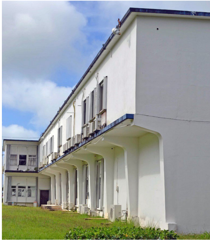
Figure 109. Feature 1, second floor office extension.
