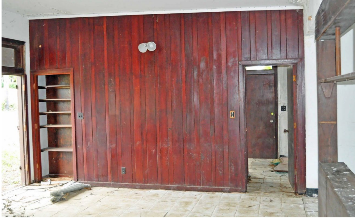
Figure 159. Feature 50. Tongue and groove wall separating living room from kitchen and laundry with its original stain and varnish finish. Note small closet and double light fixture which are both original.
