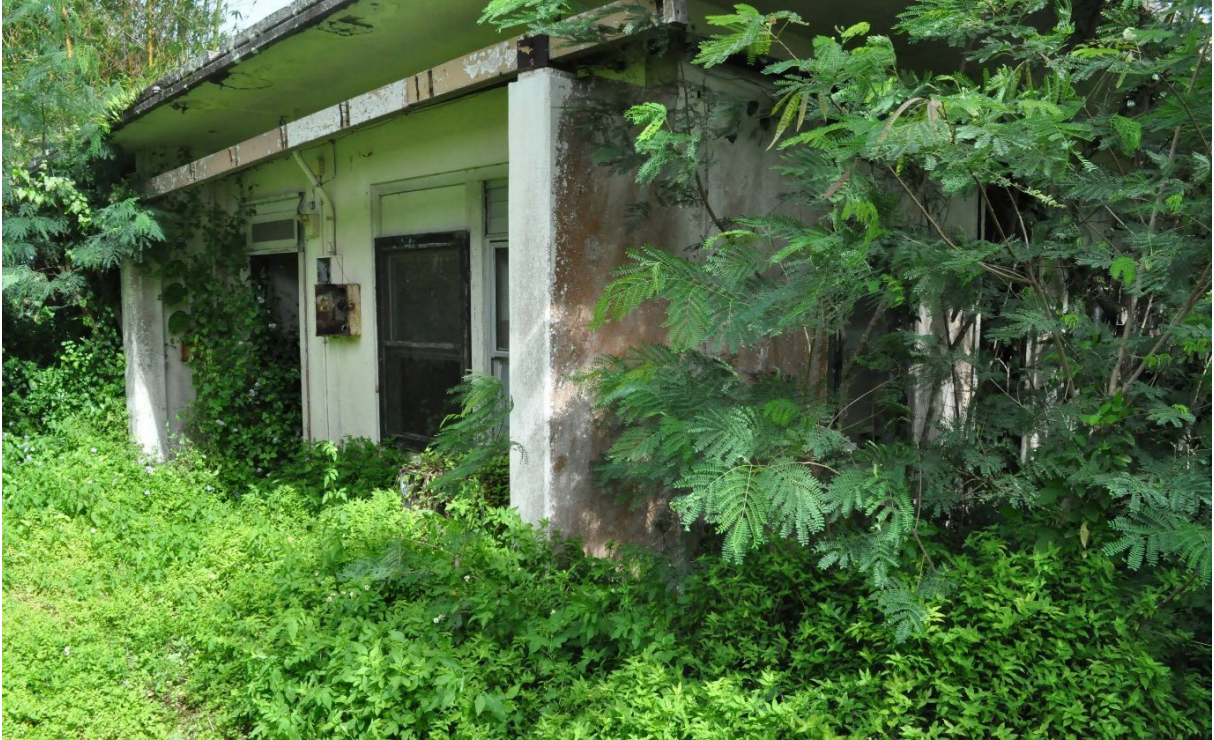
Figure 9. An abandoned former residential unit.
