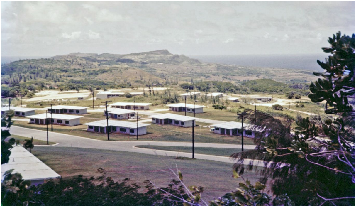
Figure 38. A view of newly completed residential units on the 1200 block. Power lines have not yet been strung. Also visible in background is the administration building, warehouses, and motor pool.
