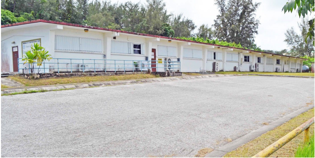
Figure 182. West and north elevation views of Feature 75 showing tapered vertical and horizontal support members. Feature 76, the original dispensary parking lot, is visible in foreground.
