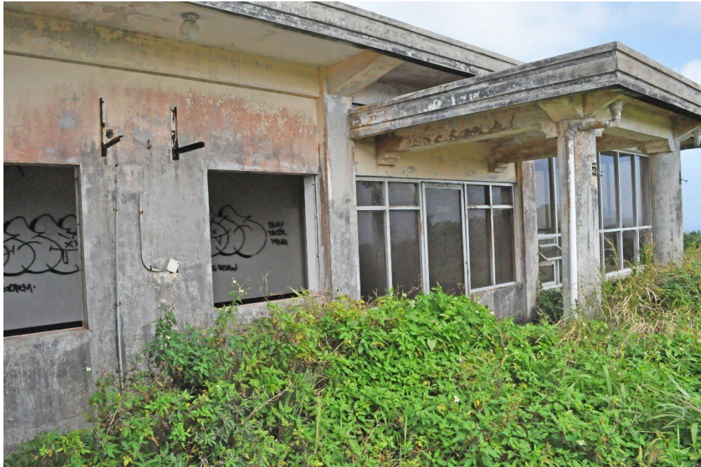
Figure 198. Feature 124 showing a concrete block extension built to house a government office in the 1990s.
