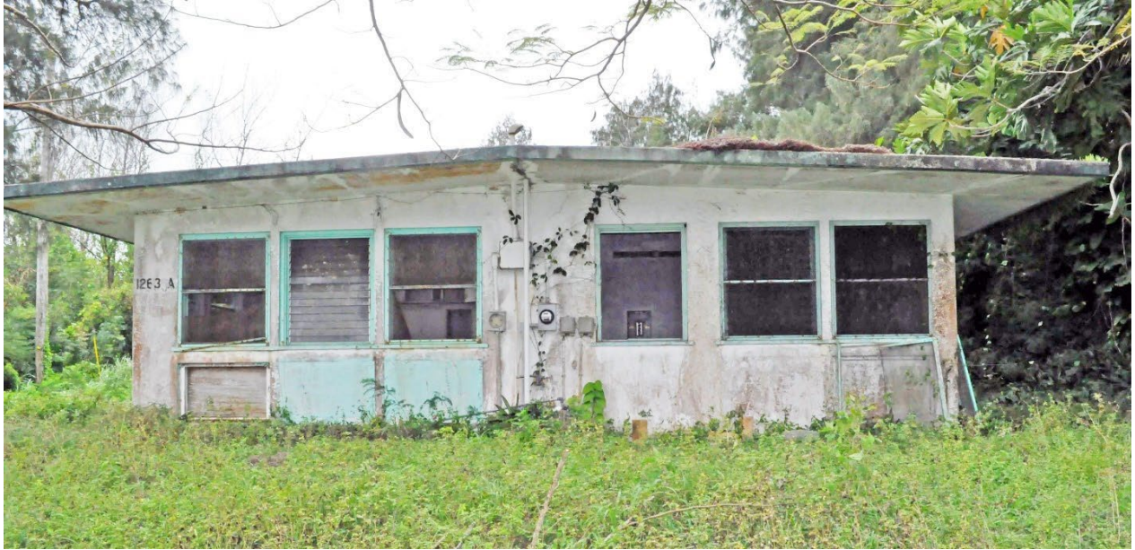
Figure 186. Entrance end of Feature 136. Original door, center right, was converted to a window.
