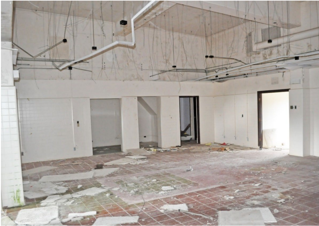
Figure 194. Kitchen of Feature 124. Note tiled walls (originally aqua blue) and wires for a modern drop ceiling.
