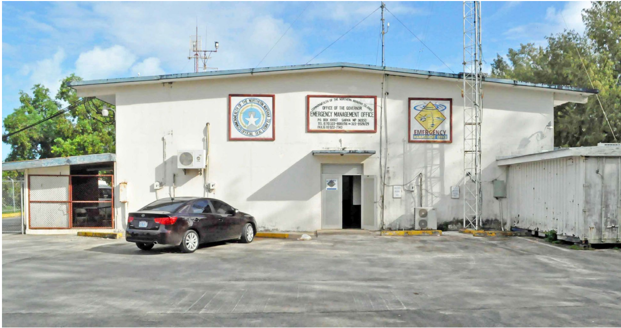
Figure 175. South elevation of Feature 71. The parking area is not an original feature.
