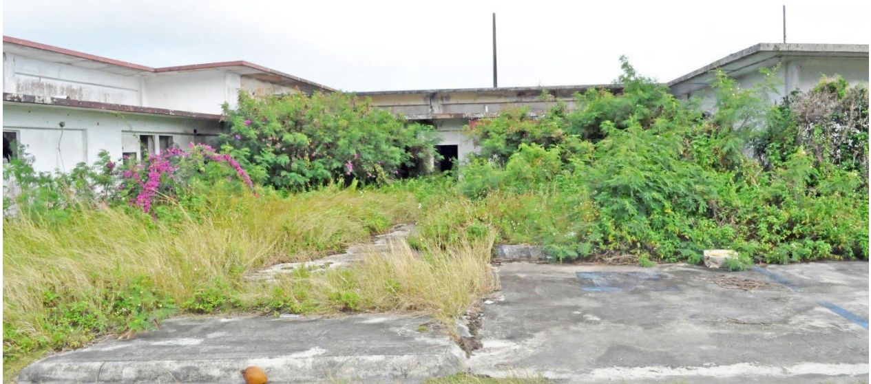
Figure 191. Feature 124 south elevation view. This building is abandoned and overgrown in vegetation that obscures the original main entrance doors.
