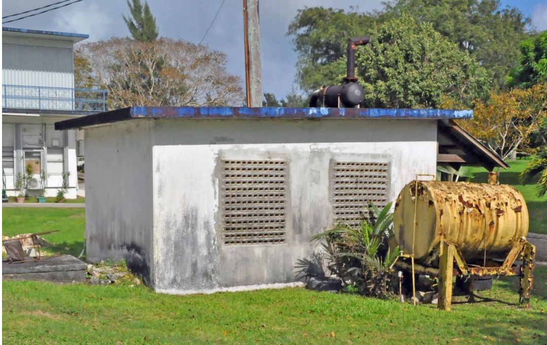
Figure 117. Original NTTU generator building, Feature 3. Old fuel tank at right.
