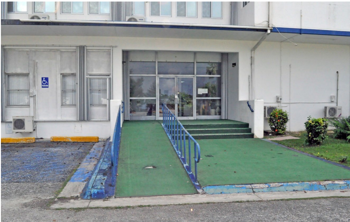
Figure 106. Main entrance to Feature 1. Note wheelchair ramp that was added during 1987 renovation work.
