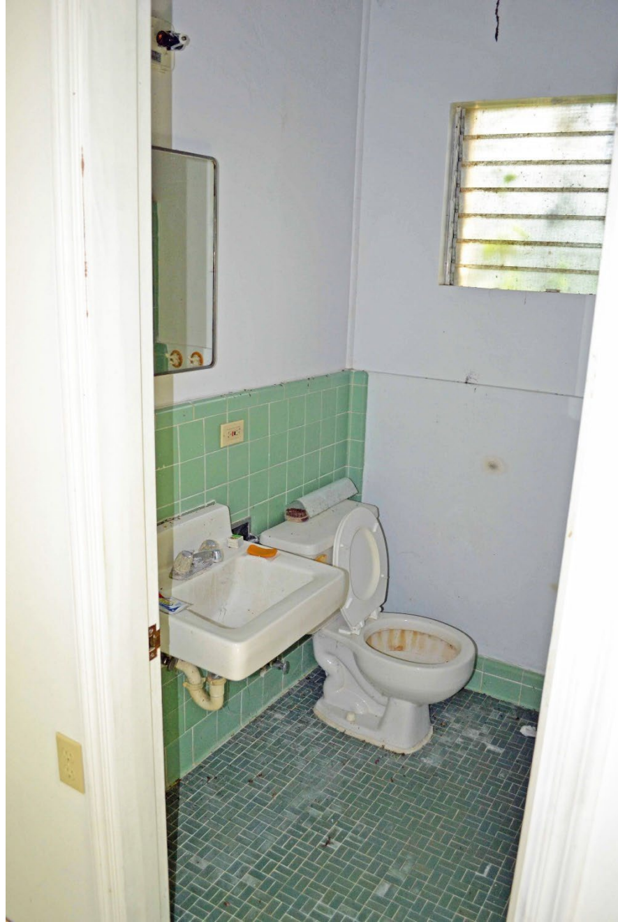
Figure 163. MOQ, Senior (Feature 65). Master bathroom details. Also present is a shower stall at right. Wall tiling suggests that the bathroom was originally fitted with a large pane and louver window. The original window was modified by covering the lower half with plywood and inserting a smaller window with glass louvers (of the kind popularly used in the 197s and 80s). The size of the lower portion of the original window is delineated by the green edging tile.
