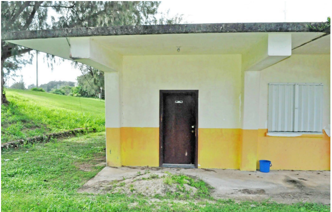
Figure 177. Feature 71, low wing detail. Note tapered vertical and horizontal support elements and wide roof overhang.
