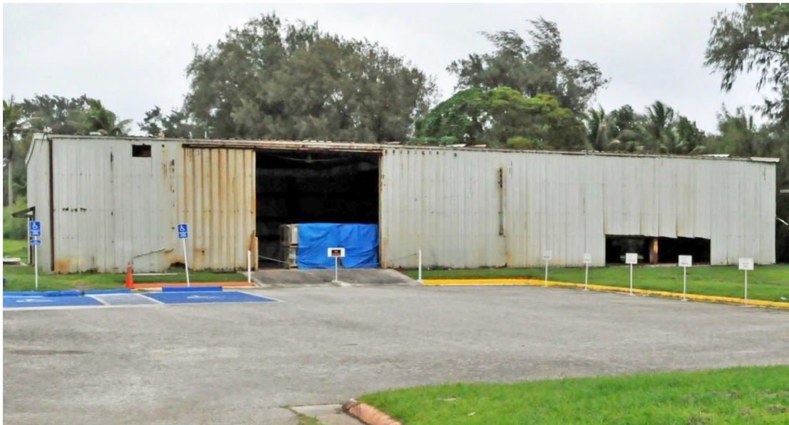
Figure 140. Feature 14. This steel “Butler” style warehouse was built by the TTPI government sometime after 1969. It was subsequently demolished after the 2011 survey. Only its concrete slab is extant.
