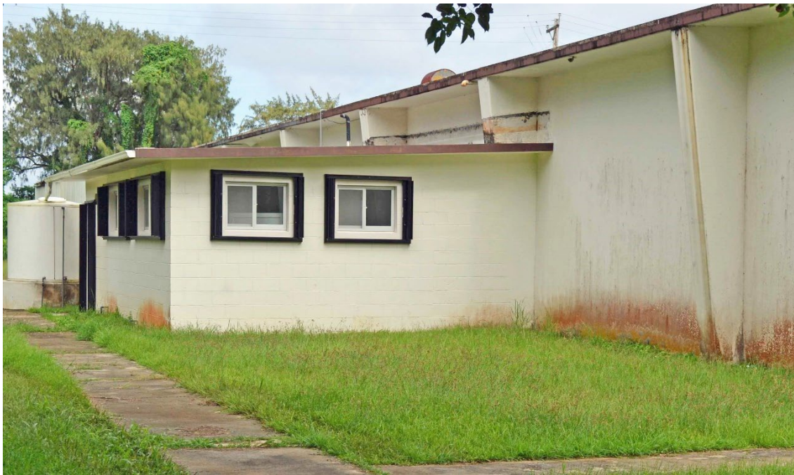
Figure 138. Concrete block extension on west elevation of Feature 11a built in the early 1970s.
