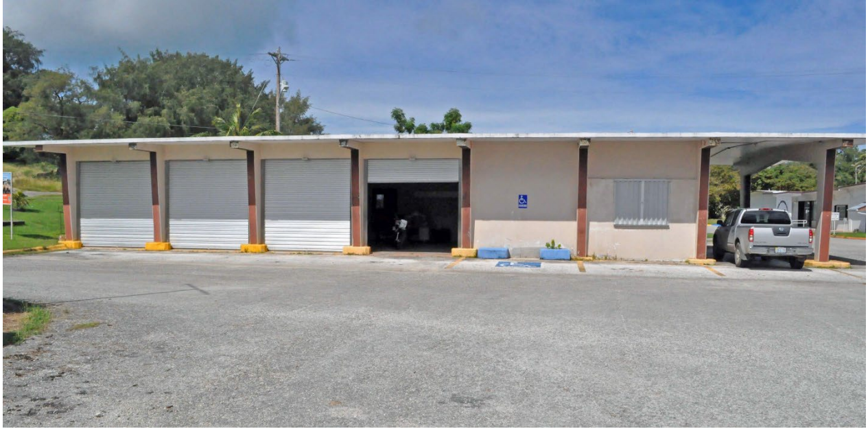
Figure 121. Feature 6. Looking west. Note that northernmost service bay has been walled off.
