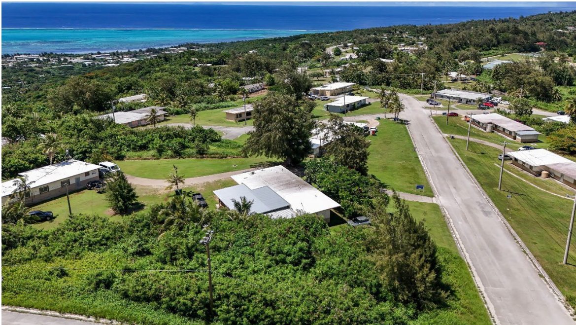
Figure 8. A current view of the 1200 block showing the proliferation of vegetation.
