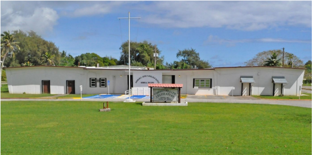
Figure 133. Feature 11a-c. The original dehumidified and general warehouses were made a single building in the early 1970s with the addition of central office space. The two original NTTU warehouses (Features 11a and b) can be seen at either end of the combined building. The building is now occupied by the CNMI legislature.
