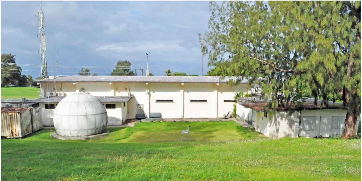
Figure 176. East elevation of Feature 71 showing the “multi-purpose” room at left and a portion of the “low wing.” The original large windows in the multi-purpose room have been closed. Note concrete block extension at far left
