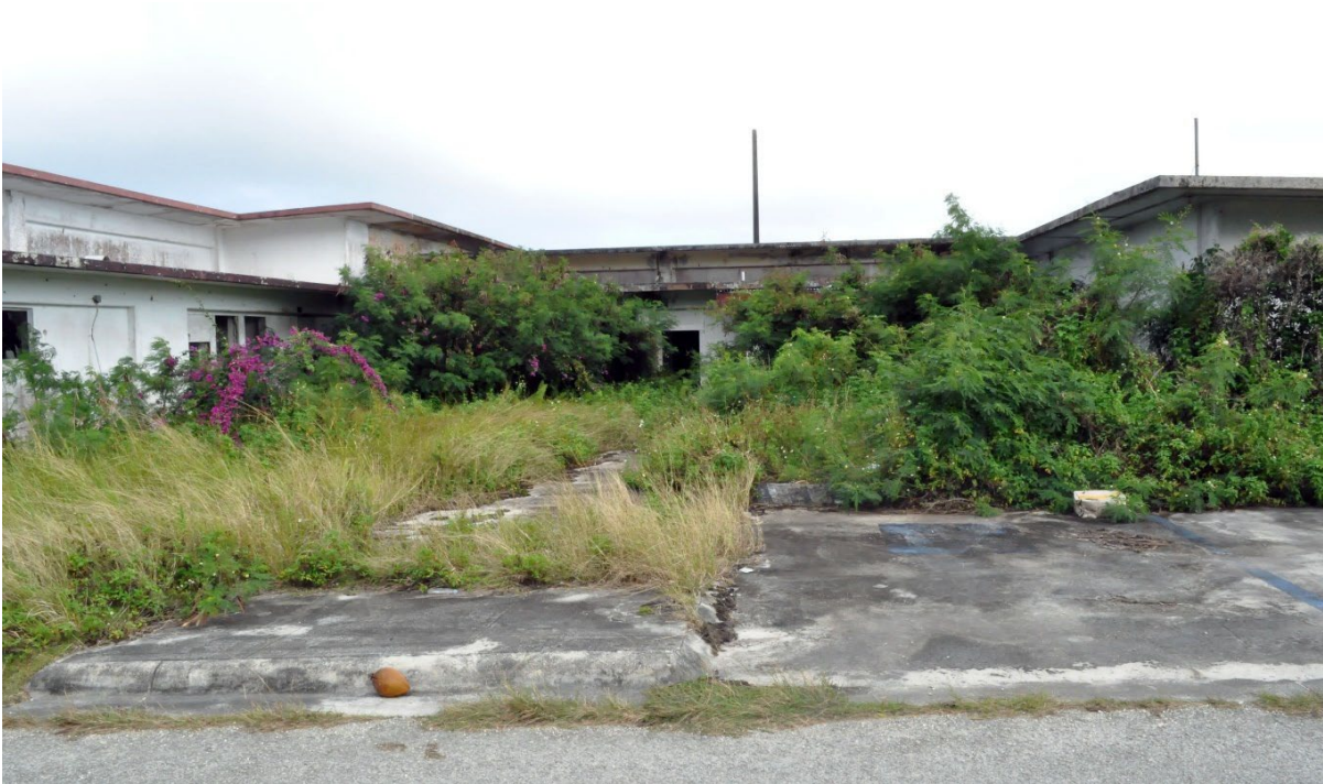
Figure 10. The former mess/club building now abandoned and overgrown in vegetation.
