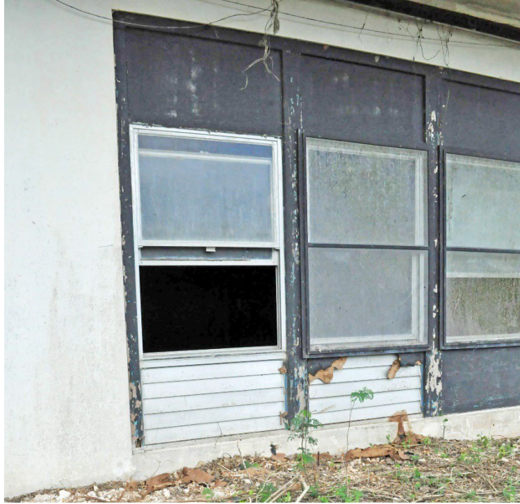
Figure 155. Feature 50 with original sliding pane windows and lower aluminum louvers. Upper louvers are also present.
