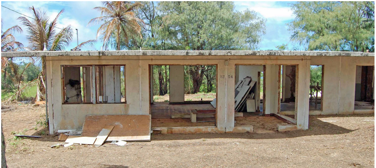
Figure 167. MOQ, Junior (Feature 121). This unit has been stripped to its concrete shell in advance of renovation.
