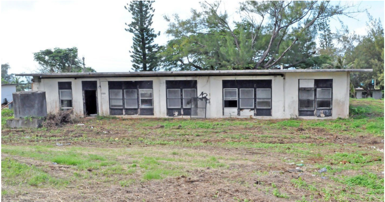
Figure 151. A MOQ, Junior in the 1300 block (Feature 50). This was the best-preserved example of this feature type documented by the survey. Note original pane windows. Original aluminum louvers are present above and below the panes, covered with painted plywood. This building was subsequently stripped for renovation with the loss of all original window, door and interior details.
