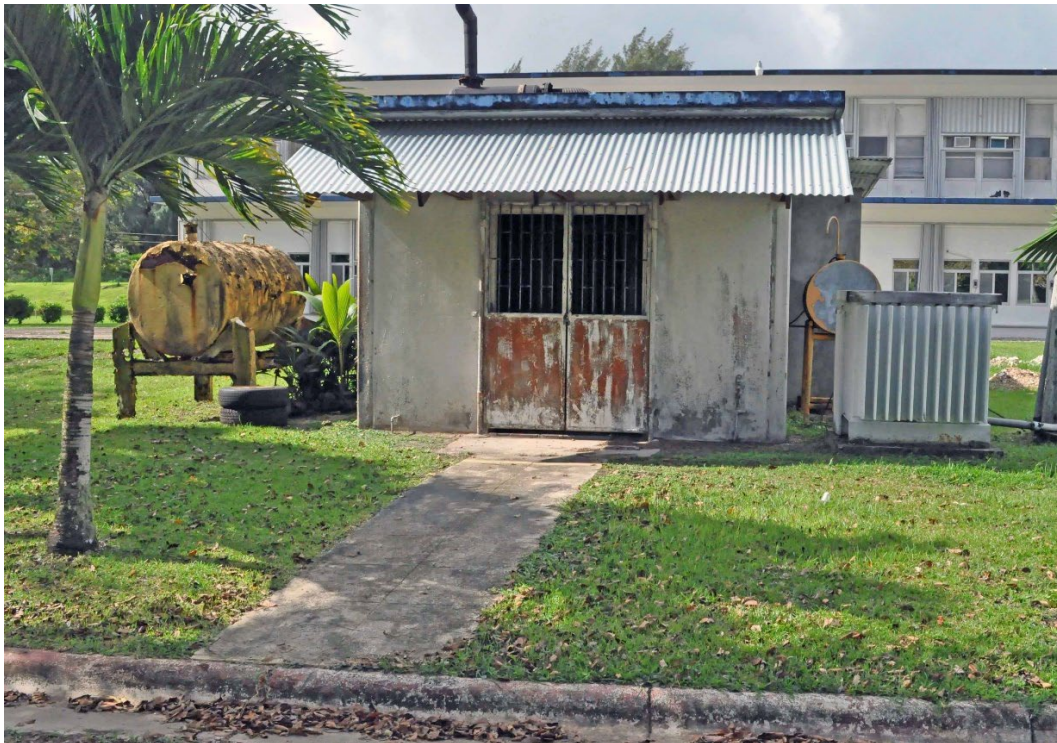
Figure 118. Main entrance, Feature 3. Current fuel tank visible at right.
