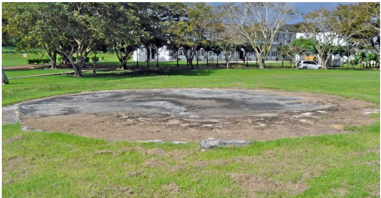
Figure 144. Feature 18. Only its concrete slab of the geodesic dome is extant.
