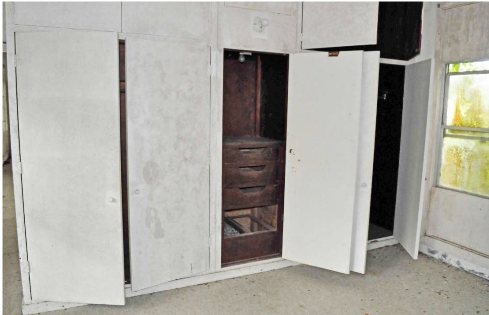
Figure 162. MOQ, Junior (Feature 128). Master bedroom cabinet details. Exterior of cabinets have been repainted white. Original dark stain finish is visible inside.
