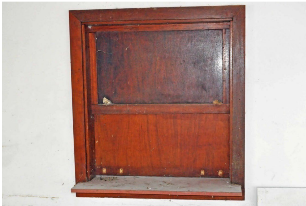
Figure 160. Feature 50. Serving window connecting kitchen with dining area. This detail possesses its original stain finish. Lifting handles have been removed but the original screw holes remain.
