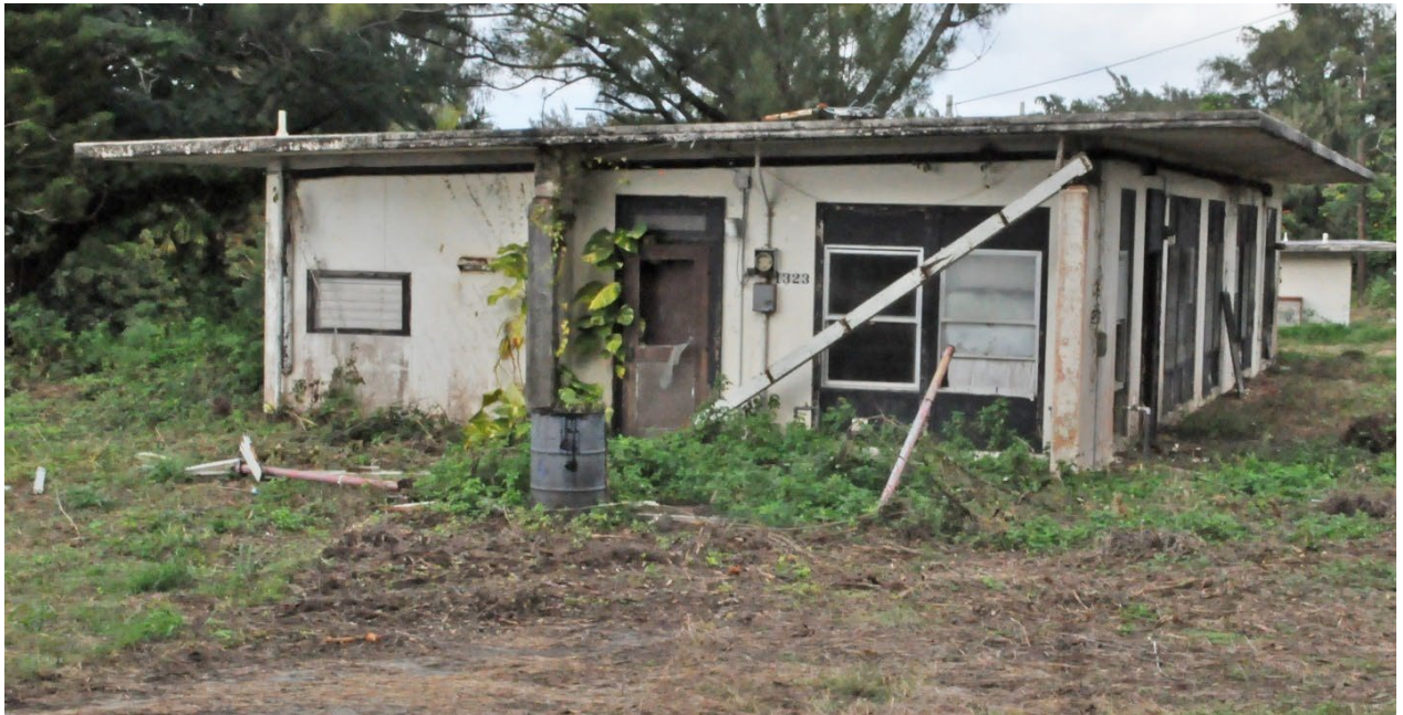
Figure 152. Feature 50 kitchen entrance. Not sloping, flat-slab roof. Kitchen on left side with utility area and half-bath to right. Hot water line with original black insulation is visible running just below roof slab. Kitchen door appears to have its original frame with a louver area above door.
