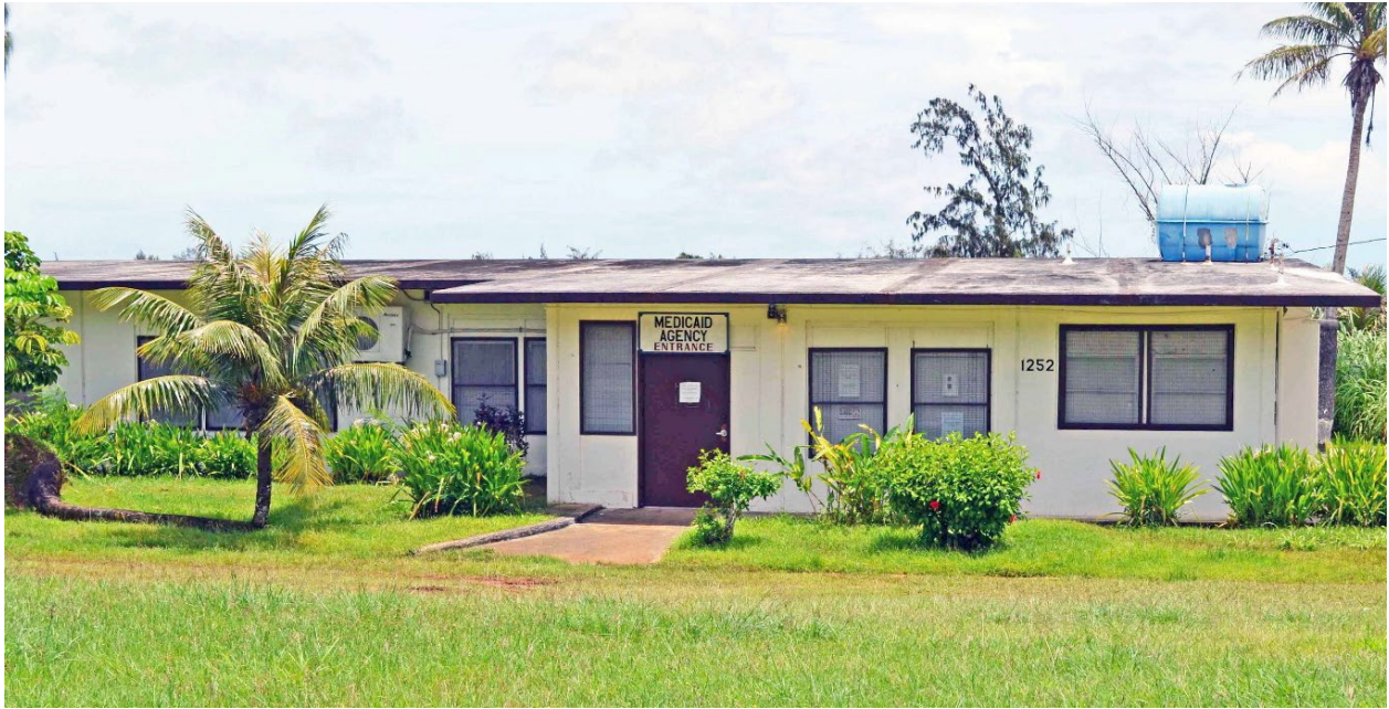
Figure 166. MOQ, Junior (Feature 123). This unit was renovated to serve as office space with minimal changes.
