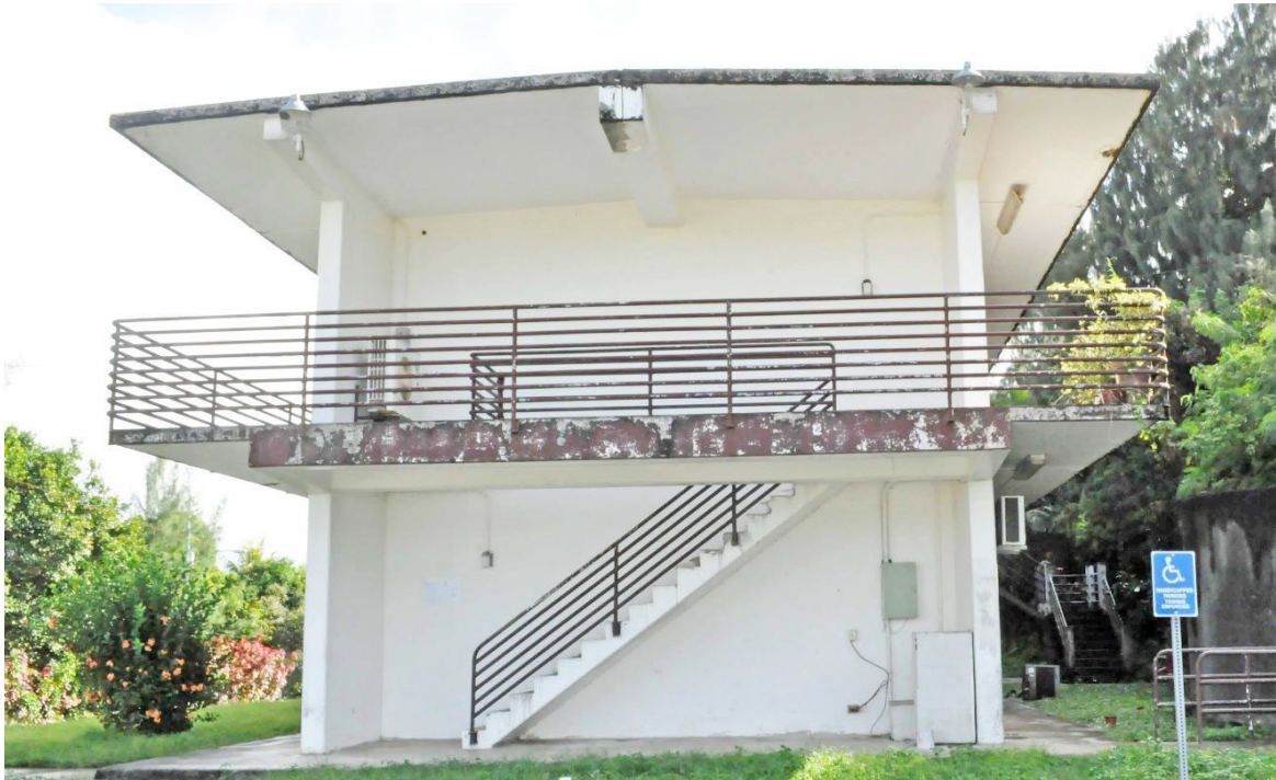
Figure 203. North elevation view of Feature 127 showing steps to second floor, tapered support elements, and low-slope gable roof with substantial overhang. Railing is not original
