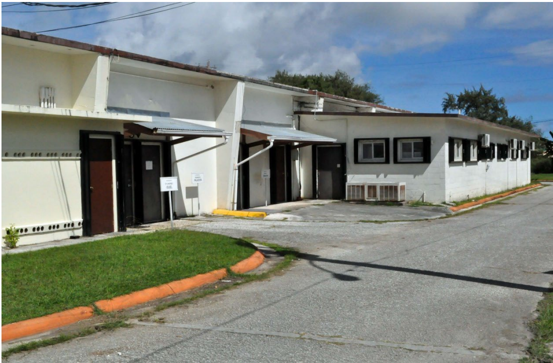
Figure 134. East elevation of Feature 11b showing concrete block extension added in the 1970s.
