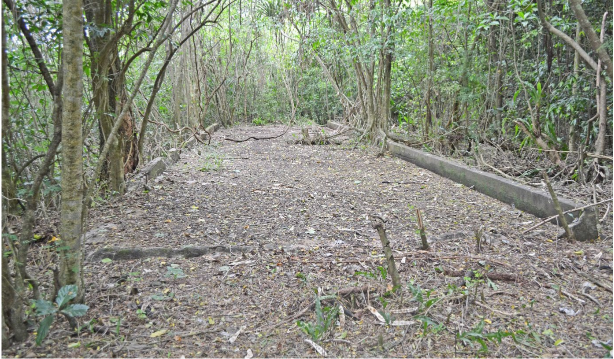
Figure 206. Bunkhouse slab in Marpi. Its wood and tin superstructure is no longer extant.
