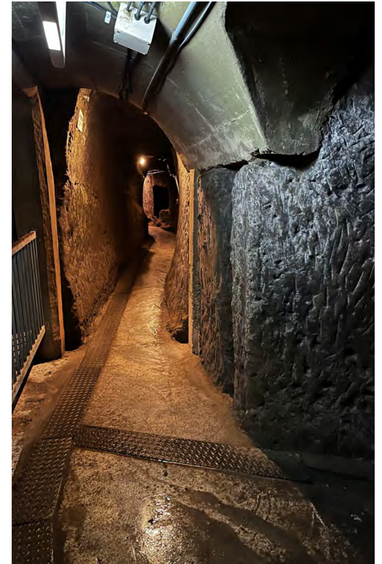
Fig. 30. The tunnel walls in the Former Japanese Navy Underground Headquarters retain signatures of the labor that was needed to excavated them.
