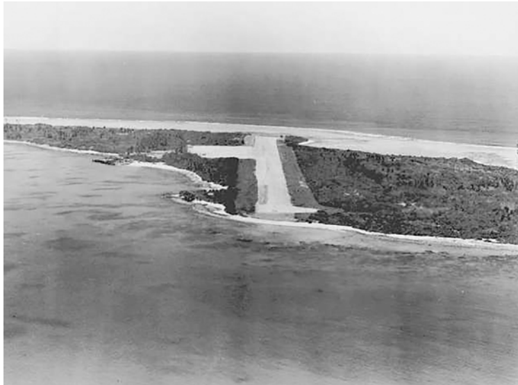
Fig. 8. (Above) U.S. military constructing an airport on Takatik Island, Pohnpei. Fig. 9. (Below) A U.S.-built airfield on Bikini Atoll completely bisecting an island.
