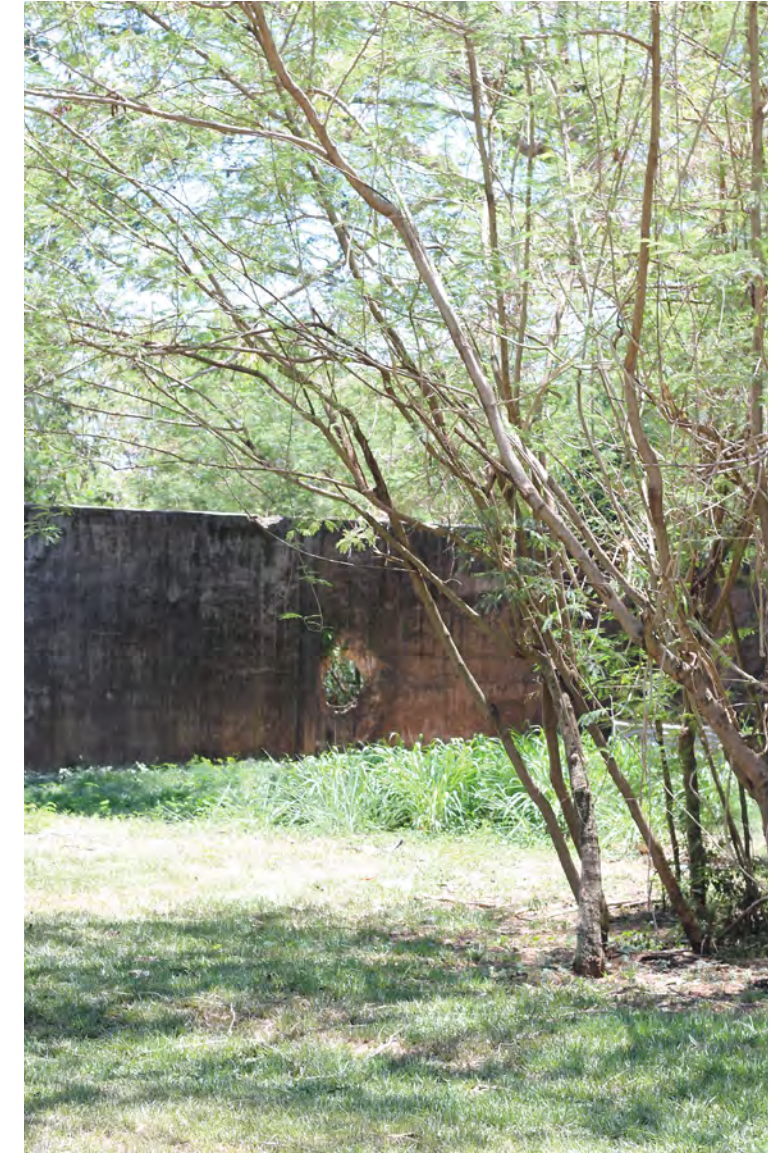
Fig. 23. Tangantangan grows freely at the Japanese Jail, often reaching tall heights with a wide spread from its multistem nature. View of inner courtyard with perimeter wall in the background.
