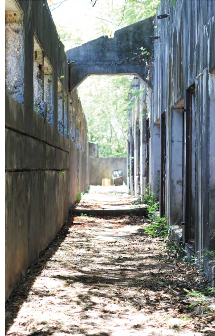
Fig. 22. A view down the longest of the three ruins still standing at the Japanese Jail, with cell doors to the right and a wall with small windows facing into the main courtyard of the Jail to the left.
