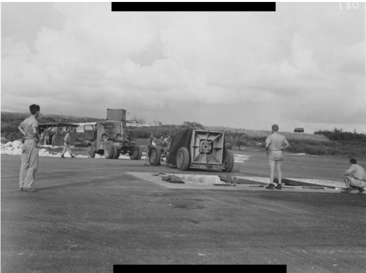
Fig. 31. (Above, right) B-29 Superfortresses fly over Runway No. 3 during buildout. Fig. 33. (Below, right) Loading the atomic bomb pits on Tinian, 1945.
