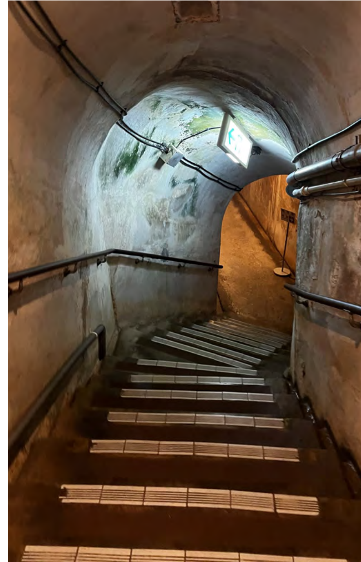
Fig. 42. Descending stairs leading into the tunnels.
