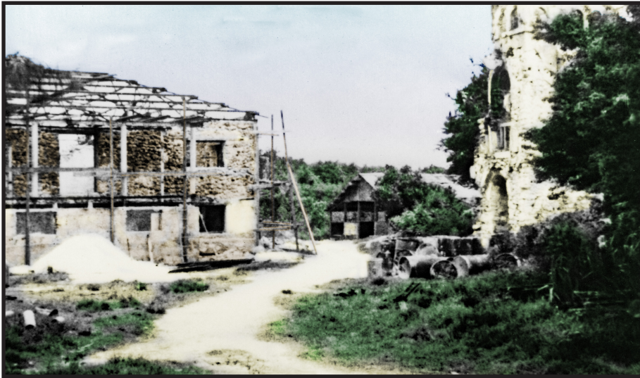
Building of the convent and rectory.
