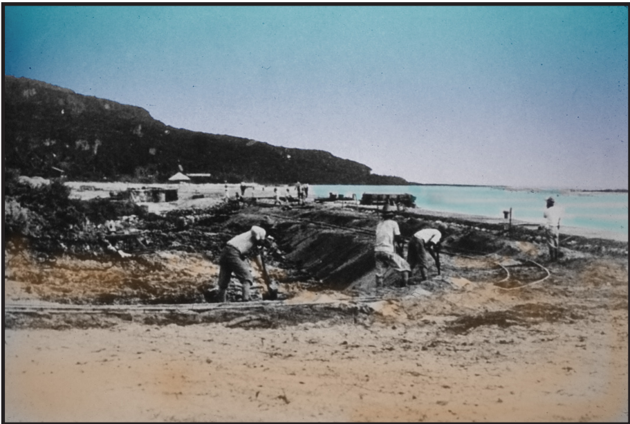
Construction of the railroad.
